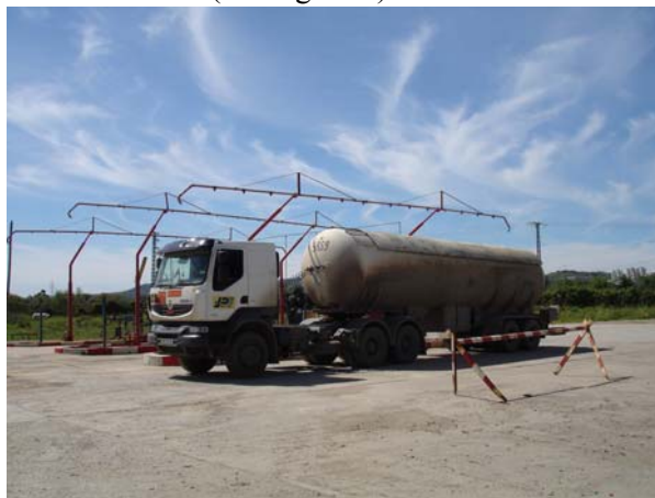
Fig. 3 – Bulk loading area.
